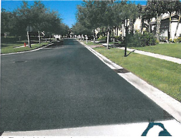
1. Typical inlets and gutters.
