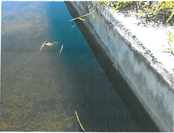
7. LWDD L-17 Canal bottom silt and weed at outfall pipe. (Outfall pipe in headwall obscured)
